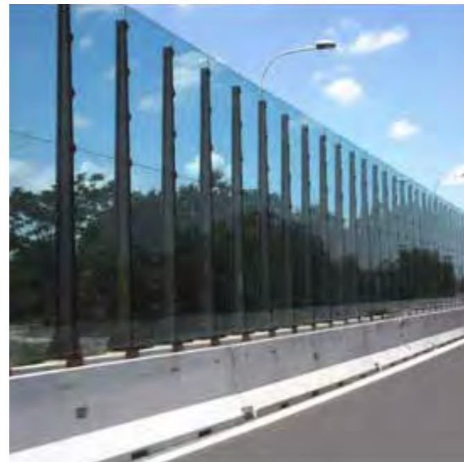
Use of transparent panels for noise barriers, integrated with parapet ©Boscoltalia
