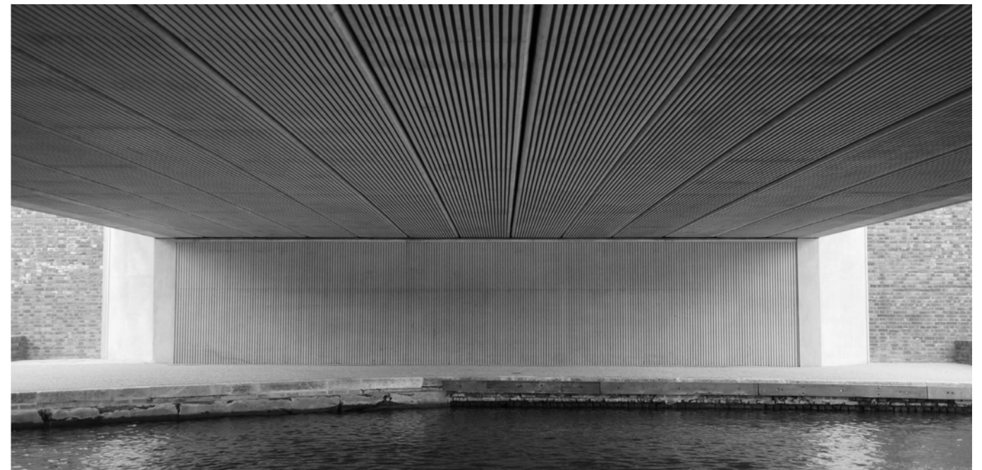
Ribbed bridge soffit, Kings Cross - texture and shadow visually reduce bulk of soffit ©KnightArchitects
