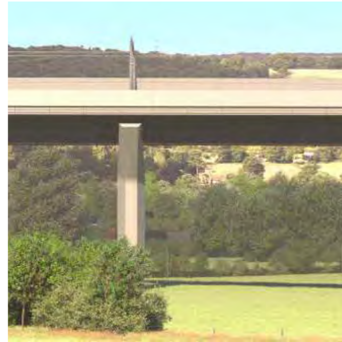
Shadow and materials create visually reduced deck depth ©HS2
