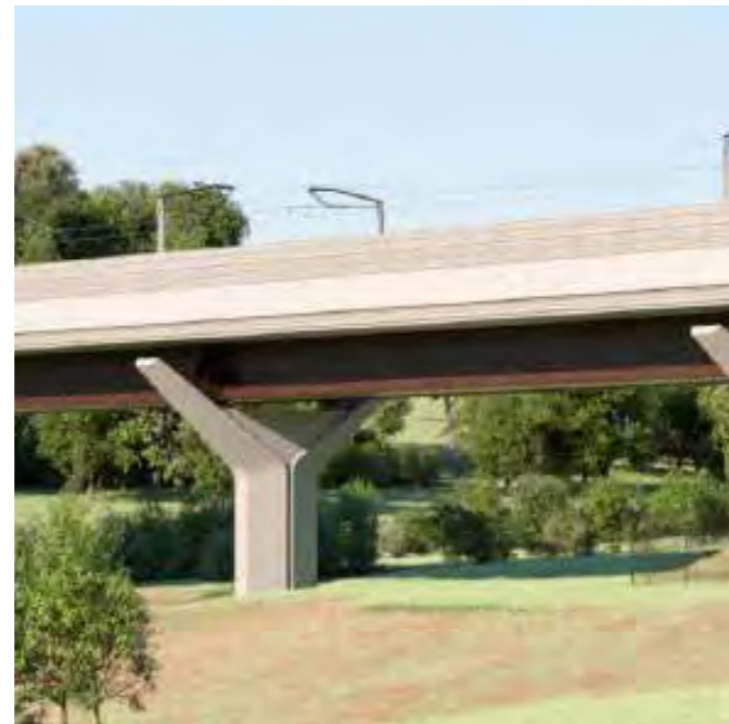
Exposed crossheads interrupt the viaduct soffit creating rhythm. Deck soffit colour and shadow reduces depth ©HS2
