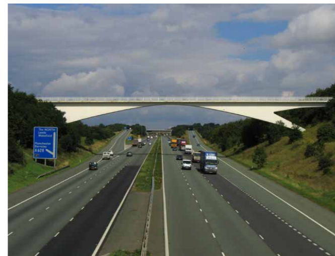
Single span overbridge with distinctive piers and planting to visually break up bulk and integrate with adjacent planting. ©Klauswithk
