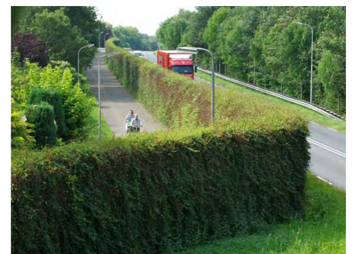
Green noise barriers © BAMWegen
