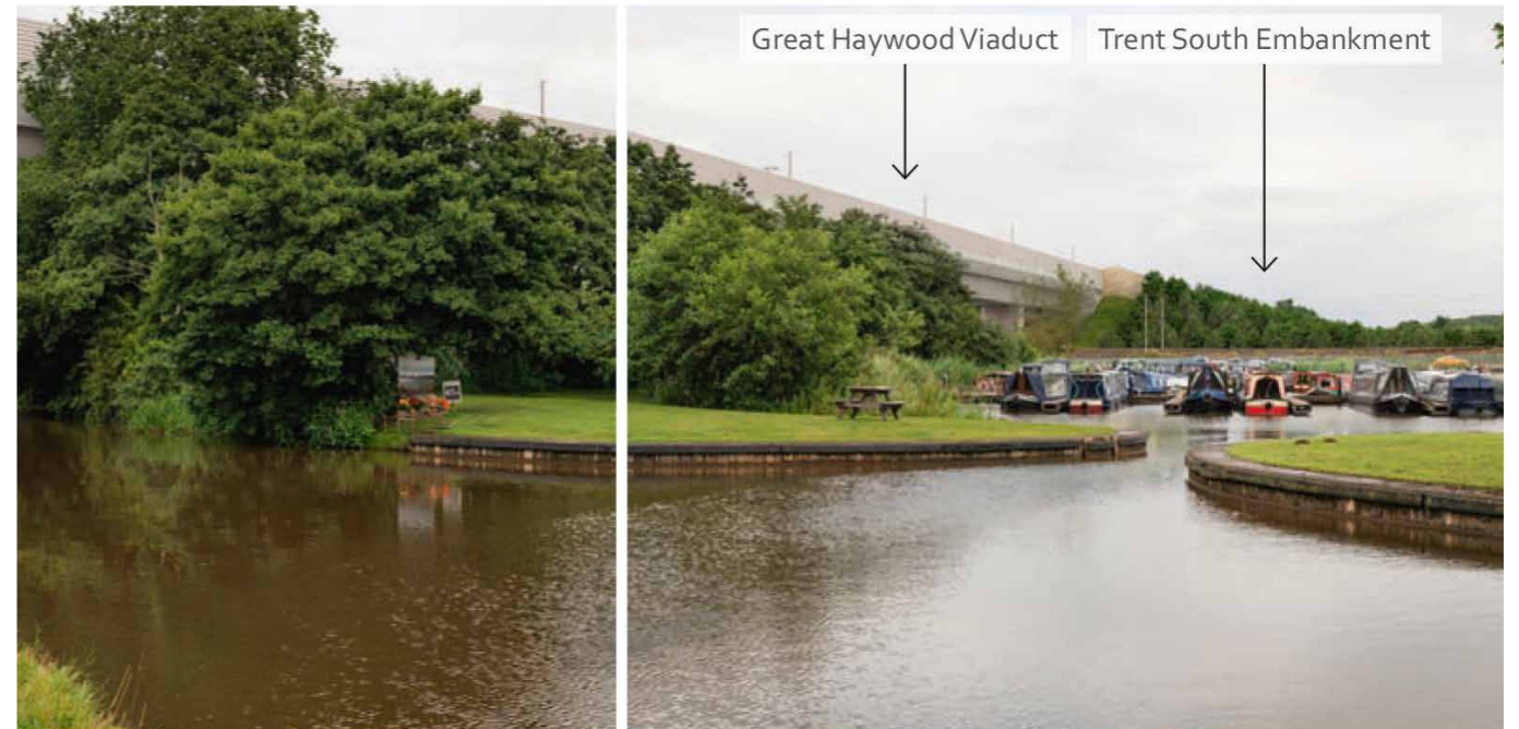
View north along Trent and Mersey Canal Towpath adjacent to marina (Viewpoint 0009.03.007 from LV-01-636) ©HS2
