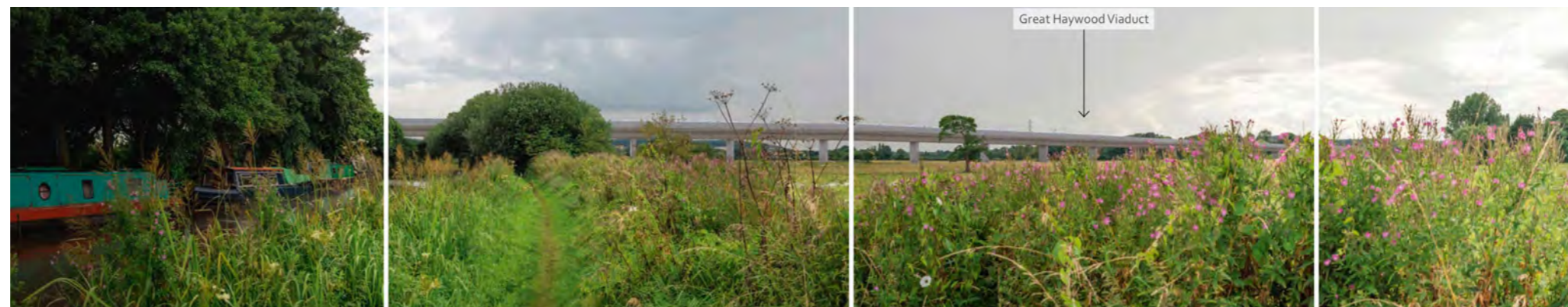
View south west along Trent Mersey Canal towpath towards proposed Great Haywood Viaduct (Viewpoint 009.03.021 from LV-01-658) ©HS2
