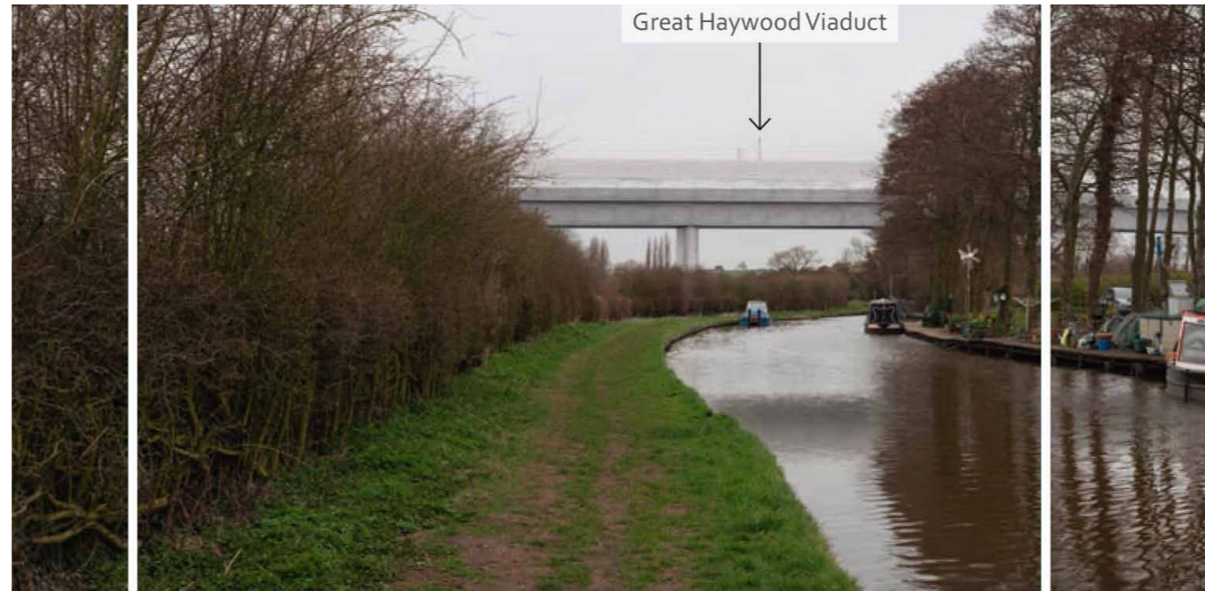
View north along Trent and Mersey Canal Towpath adjacent to marina (LV-01-524) ©HS2
