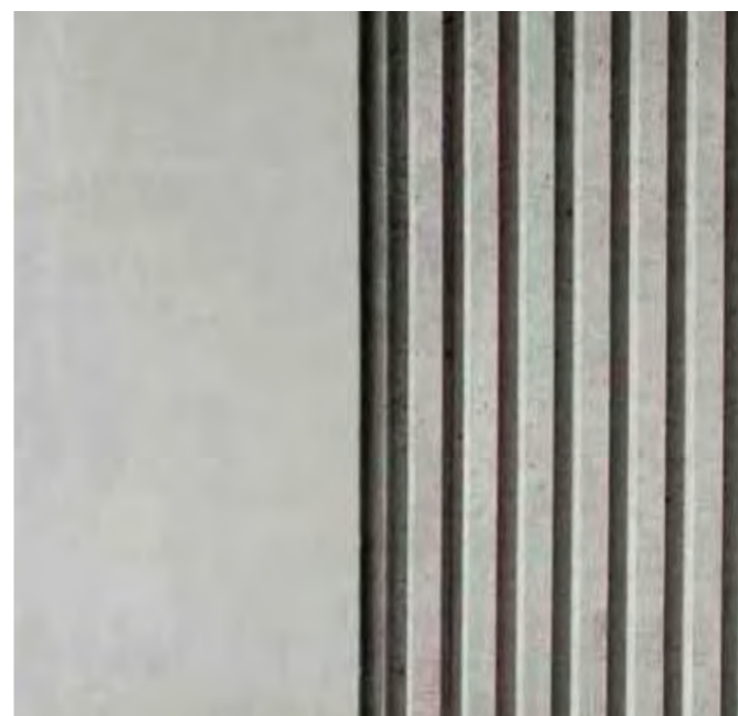
Texture and shadow gaps mask joints and reduce mass of structures ©CRT
