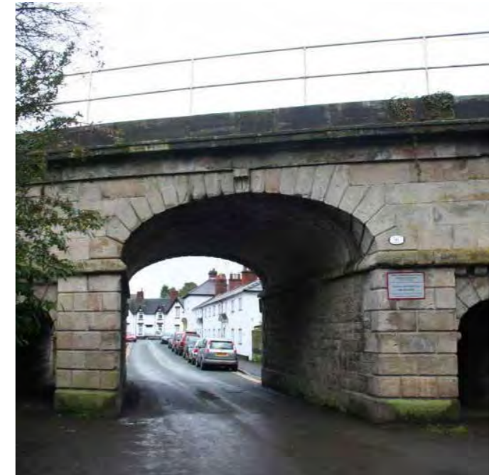
Railway bridge over Trent Lane creates a gateway into Great Haywood ©BritishListedBuildings
