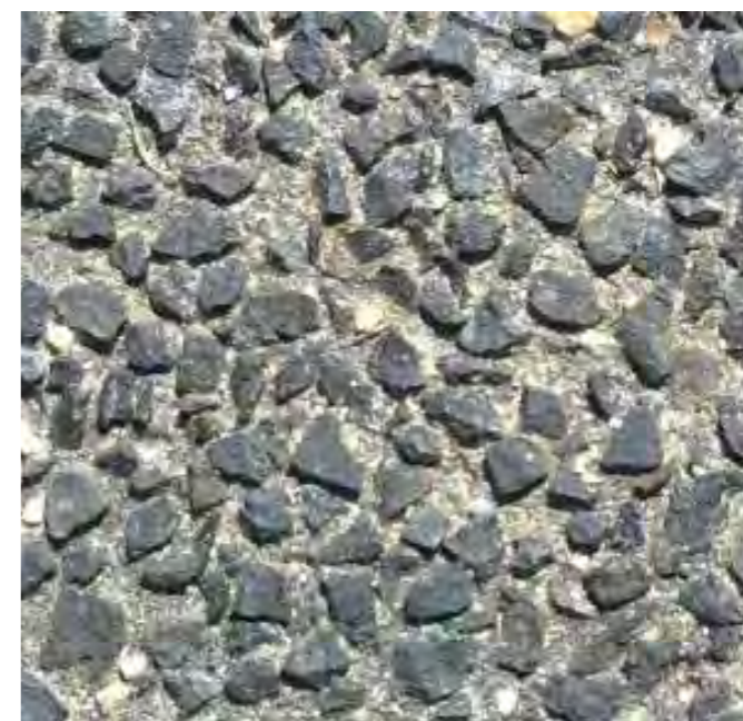
Exposed dark coloured exposed aggregate concrete
