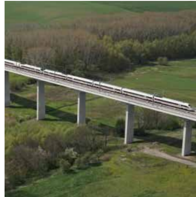
Scherkondetal railway viaduct near Weimar, Germany. Slender piers are elegant and piers at regular intervals allow reduced bridge deck. ©NormanHallermann
