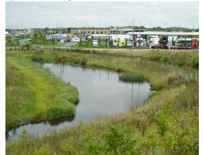
Well integrated attenuation pond, Wetherby Services ©AnthonyDixon
