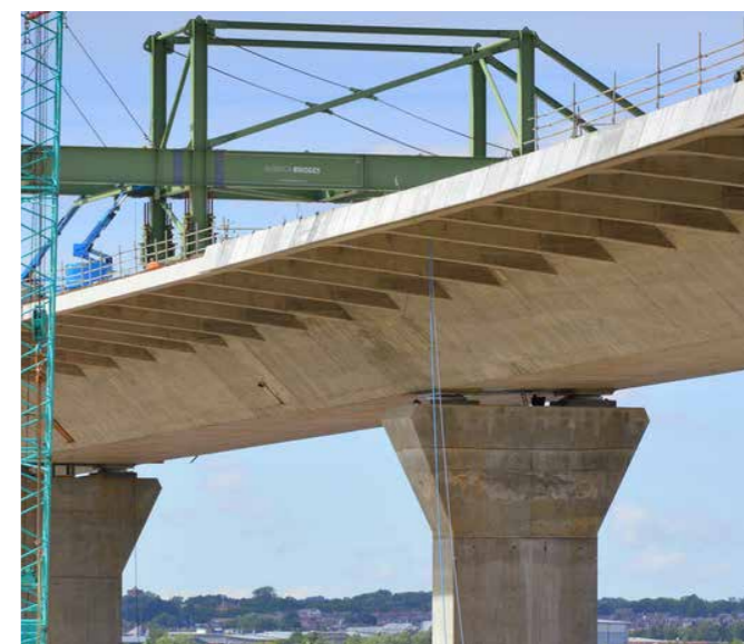
Ribbed cantilevered deck on the Mersey Gateway Bridge ©VincentPhillips
