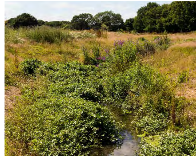
Well vegetated informal two stage channel/ ditch ©Susdrain
