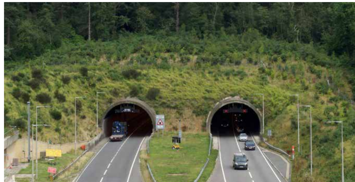
Careful slope gradients marrying into existing land form, with landscape and ecological planting in the Devil's Punch Bowl SSSI for the A3 Hindhead ©Natural England
